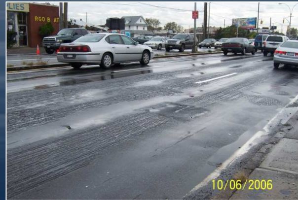
Poor Surface Drainage
