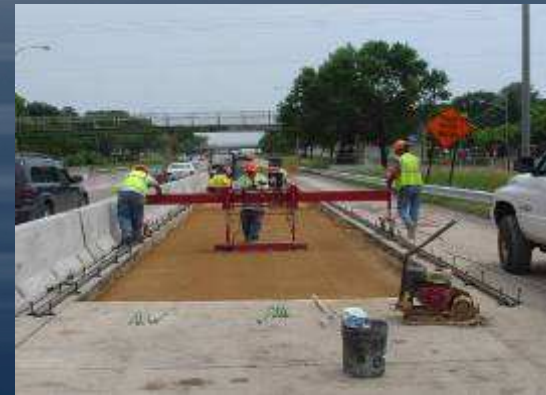
Hand Operated Grader (H.O.G.)
