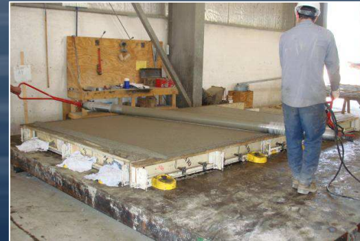
Roller Screed - Accurate Top Surface
