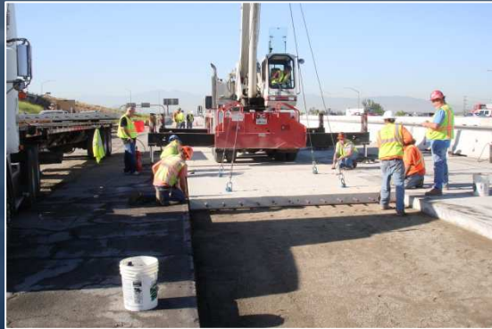
Crane Occupies New Slabs
