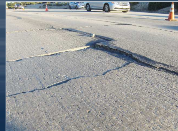
Heavily Faulted Slabs Pasadena, CA
