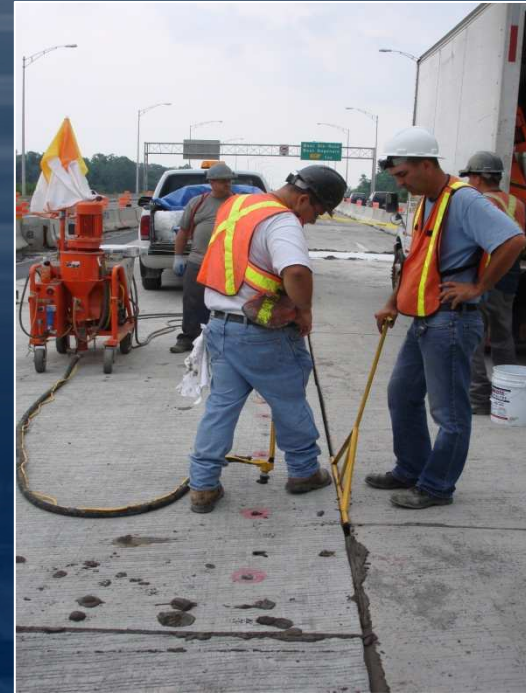
Contractor-Designed Joint Dam
