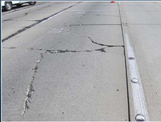
Shattered Slabs Pasadena, CA
