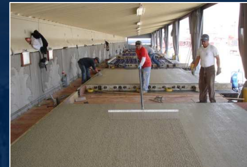
Ideal Finishing (and curing) Conditions
