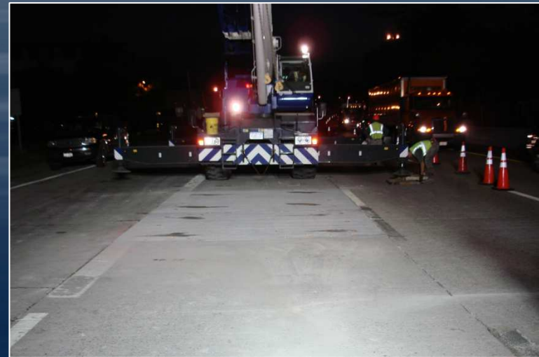
Crane Occupies New Slab
