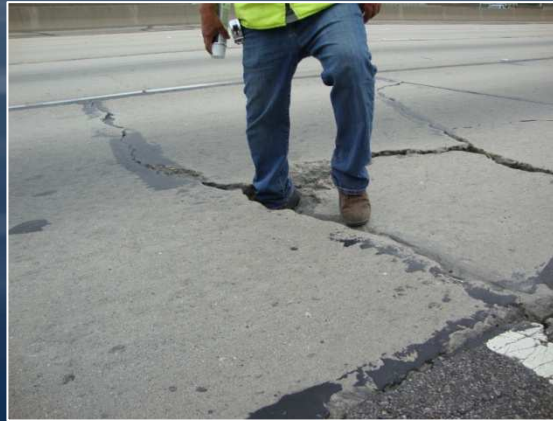
Failed Rapid Set Patches Hollywood, CA
