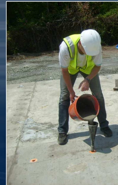
Keep Ports Full by "topping off"
